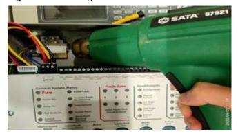
**Step 2** Take out the fuse box and replace the fuse.
