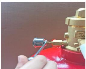
2. Use the adjustable wrench delivered with the fire cylinder to rotate the large hex nut on the valve counterclockwise until the red line is aligned (less than one circle). Ensure that the pressure gauge has readings.
