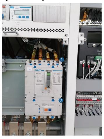
Figure 7-73 Removing the AC main switch
