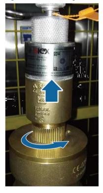
**Step 3** Loosen the fire extinguishing high-pressure hose by rotating it counterclockwise using a pipe wrench.
