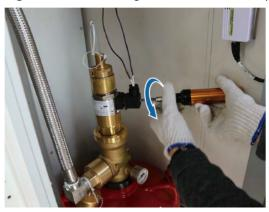
**Step 2** Rotate the solenoid valve counterclockwise to remove it from the fire cylinder.
