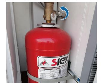
**Figure 7-84** Loosening the fire extinguishing high-pressure hose
