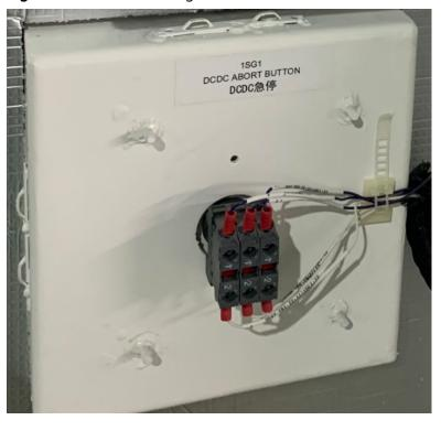
Figure 7-45 Disconnecting cables from the abort button
