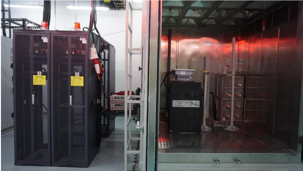
Figure 7. Photograph of test connection
