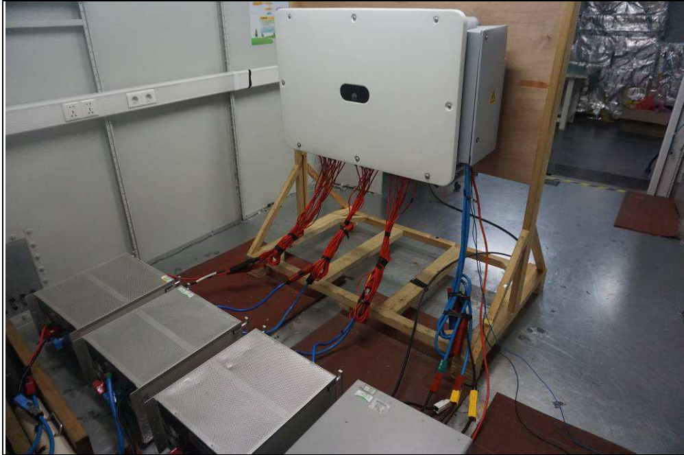
CONDUCTED EMISSION TEST (AC Power Port)
